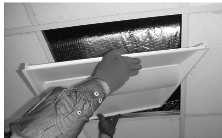
Step 5 Install troffer into grid.
