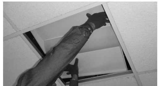
Step 6 Adjust fixture to sit properly in grid. Ensure fixture is installed based on the local codes.
