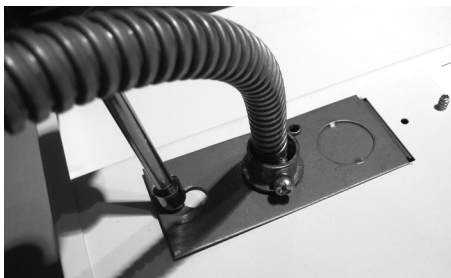
Step 4 Reinstall the knock out plate.
